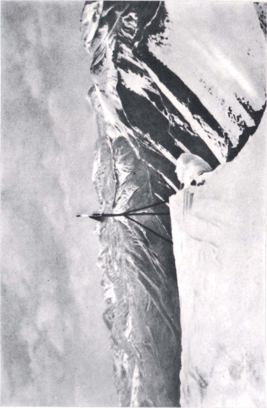
OPAQUE SIGNAL USED BY THE RUSSIAN TRIANGULATION PARTY ON THE TAGHDUMBASH FAMIR.
